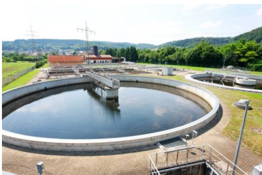
Picture 1: The municipal treatment plant in Rotenburg a. d. Fulda is designed for the equivalent of 34,000 residents and serves around
