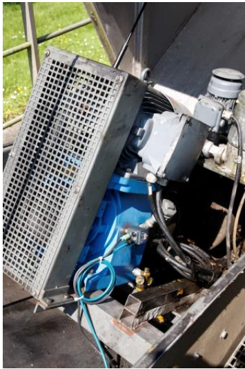
Picture 4: An intelligent FAG SmartCheck vibration sensor is attached to each of the three pump drives in the return activated sludge pumping station.
